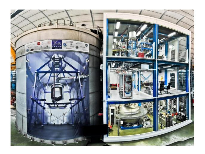
XENON1T installation in the underground hall of Laboratori Nazionali del Gran Sasso. The three story building on the right houses various auxiliary systems. The cryostat containing the LXeTPC is located inside the large water tank on th left, next to the building. Credit: Roberto Corrieri and Patrick De Perio
