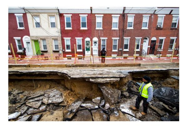
In this Jan. 9, 2017, file photo, workers inspect a sinkhole in Philadelphia. The Philadelphia Water Department said a water main break caused the sinkhole to open up on the street. Sinkholes are not a new phenomenon in the United States, but a recent spate of huge, sudden-appearing caverns is prompting alarm because they're happening in places where they were once rare. (AP Photo/Matt Rourke, File)
