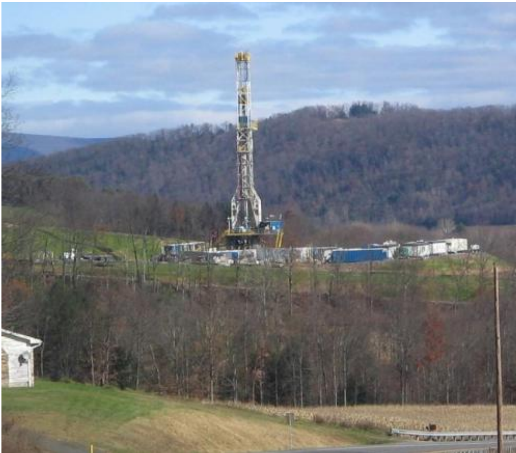
Derrick and platform of drilling gas wells in Marcellus Shale - Pennsylvania. Credit: Wikipedia/ CC BY-SA 3.0
