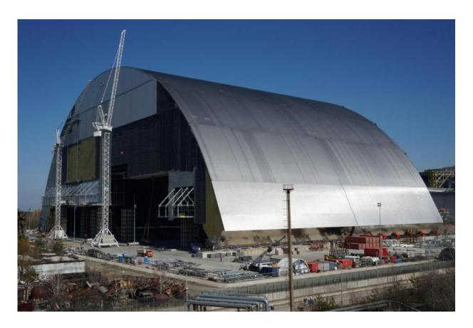
Construction of the main structure was completed in 2016. An engineering wonder, the steel arch was the largest moveable structure in the world. Credit: Pacific Northwest National Laboratory
