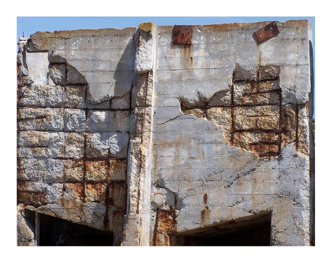
An abandoned building on Northern California's McAbee Beach shows the destructive power of corrosion on a steel-reinforced concrete structure. A new NIST evaluation method using terahertz waves can detect the early stages of corrosion on steel rebars directly through their concrete covering. Credit: With
