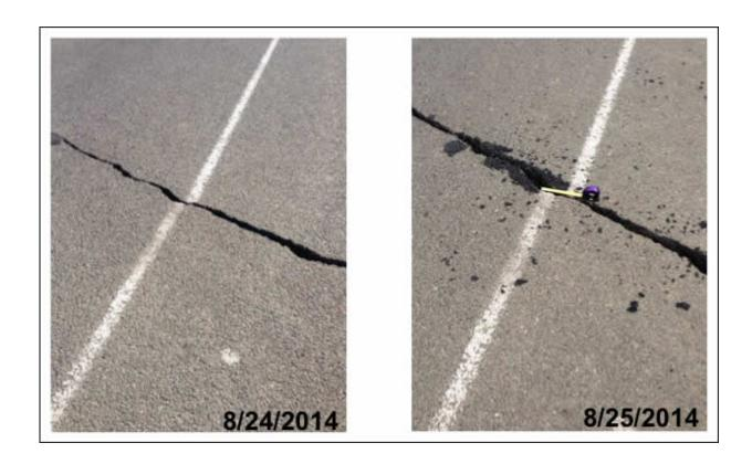
These two photos showing evidence of afterslip were taken where the West Napa fault crosses Highway 12 at Cuttings Wharf Road. The first offset measurement was taken the day of the earthquake -- about 6 cm (2 in) of right-lateral offset. The following day (almost 24 hrs later), the same feature had 11 cm (4 in) of offset. Credit: USGS/ Photos courtesy of Tim Dawson, California Geological Survey
