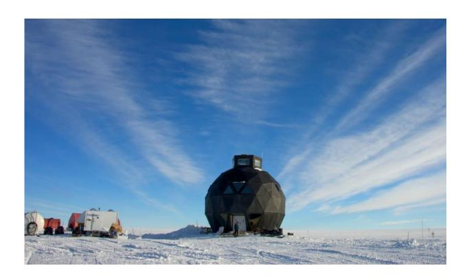
n 2015 the 14-meter high building, the 'Dome', weighing 47 tons, was pulled on skis almost 500 km over Greenland's ice-landby two tracked vehicles.
