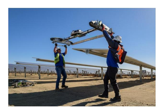
Workers at a solar station attach the robot that cleans the panels. Jobs like these are increasing rapidly as the nation moves to sustainable energy sources. Credit: L.A. Cicero
