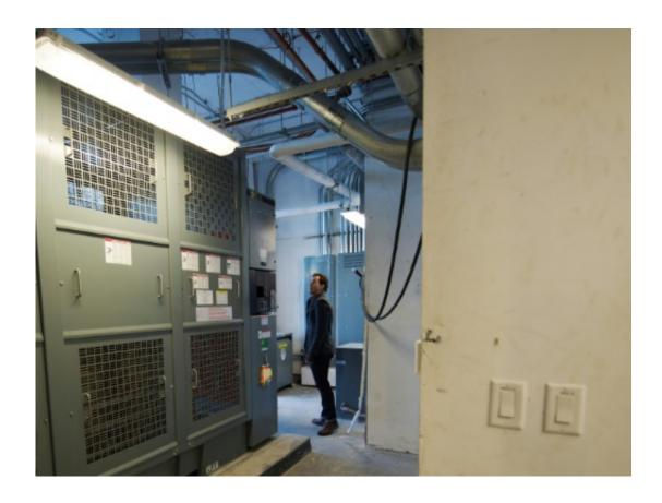
Traditionally in the basement, the heating, ventilation and large electrical equipment at the American Copper Buildings is on the first floor to minimize the risk of flooding
