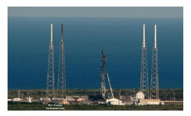
Aerial view of pad and strongback damage at SpaceX Launch Complex-40 as seen from the VAB roof on Sept. 8, 2016 after fueling test explosion destroyed the Falcon 9 rocket and AMOS-6 payload at Cape Canaveral Air Force Station, FL on Sept. 1, 2016. Credit: Ken Kremer/kenkremer.com
