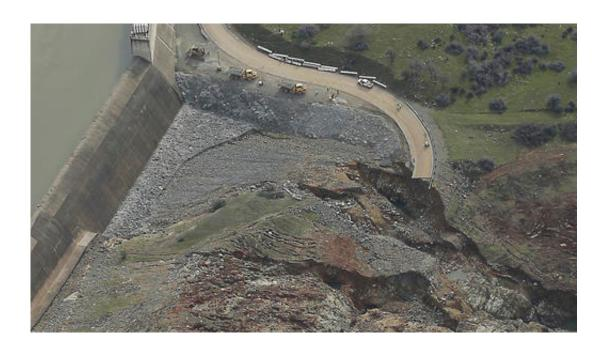
This photo taken Monday, Feb. 13, 2017, shows erosion caused when overflow water cascaded down the emergency spillway, right, of the Oroville Dam in Oroville, Calif. Water flowed over the emergency spillway Sunday morning when Lake Oroville reached capacity, and engineers determined the hillside was
