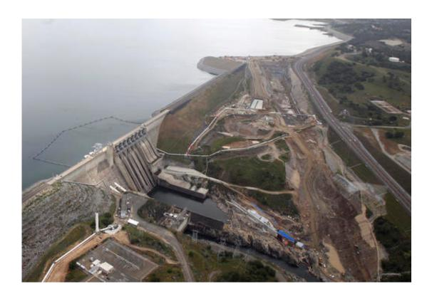
In this April 14, 2010, file photo the auxiliary spillway, right, is under construction at Folsom Dam, in Folsom, Calif. Twelve years ago, widespread destruction from Hurricane Katrina on the Gulf Coast helped compel federal engineers to spend nearly \$1 billion constructing the auxiliary spillway at Folsom Dam, scheduled to be completed in 2017. (AP Photo/Rich Pedroncelli, File)
