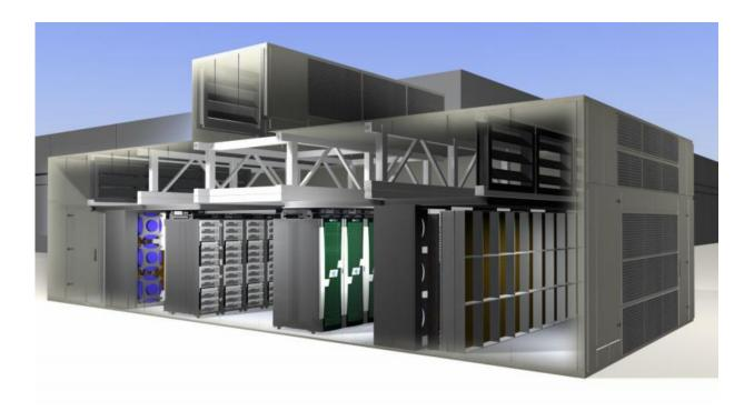
(Artist concept, interior) The Modular Supercomputing Facility (MSF) at Ames uses fan technology that consumes less than 10% of the energy used by mechanical refrigeration in traditional supercomputing centers. Credit: NASA/Marco Librero
