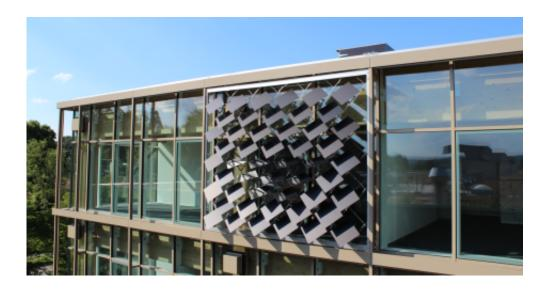
Adaptive Solar Facade. Credit: Chair for Architecture and Building Systems, Institute of Technology in Architecture, ETH Zurich
