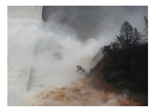
Water flows through break in the wall of the Oroville Dam spillway, Thursday, Feb. 9, 2017, in Oroville, Calif. The torrent chewed up trees and soil alongside the concrete spillway before rejoining the main channel below. Engineers don't know what caused what state Department of Water Resources spokesman Eric See called a "massive" cave-in that is expected to keep growing until it reaches bedrock. (AP Photo/Rich Pedroncelli)
