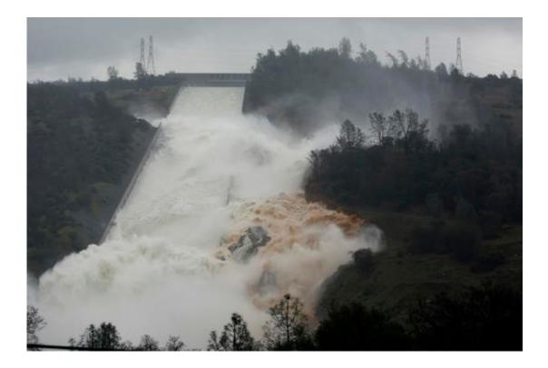
Water flows through break in the wall of the Oroville Dam spillway, Thursday, Feb. 9, 2017, in Oroville, Calif. The torrent chewed up trees and soil alongside the concrete spillway before rejoining the main channel below. Engineers don't know what caused what state Department of Water Resources spokesman Eric See called a "massive" cave-in that is expected to keep growing until it reaches bedrock. (AP Photo/Rich Pedroncelli)
