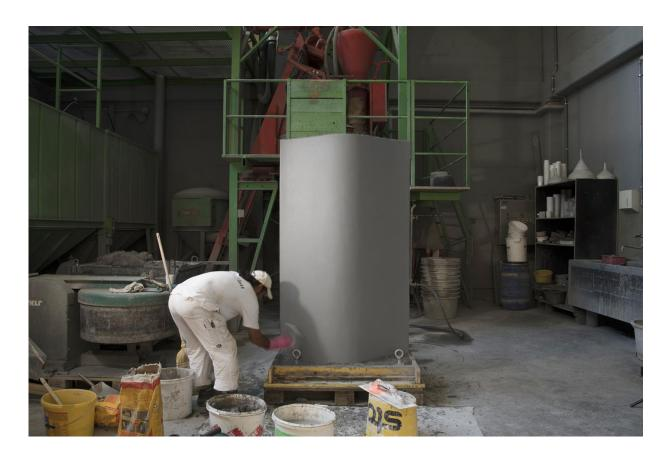
The finish of a two meter high, concrete-filled mesh prototype produced by In-Situ Fabricator construction robot. Credit: NCCR Digital Fabrication and ETH Zurich
