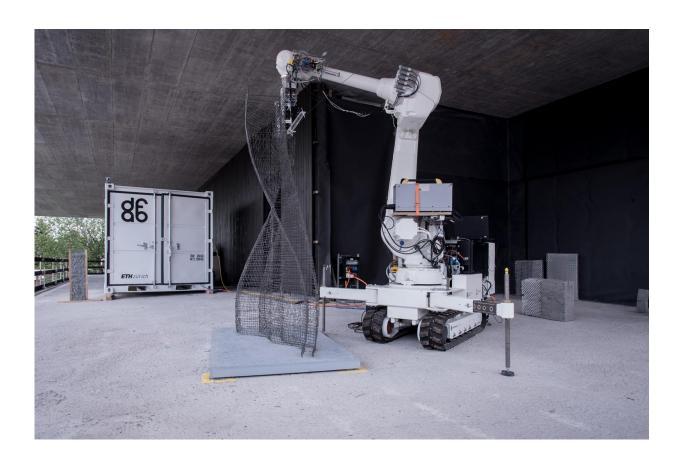
In situ Fabricator (construction robot) is fabricating a doubly curved mesh structure during a fabrication test on the Empa NEST building in Duebendorf, Switzerland. Credit: Photo: NCCR Digital Fabrication and ETH Zurich
