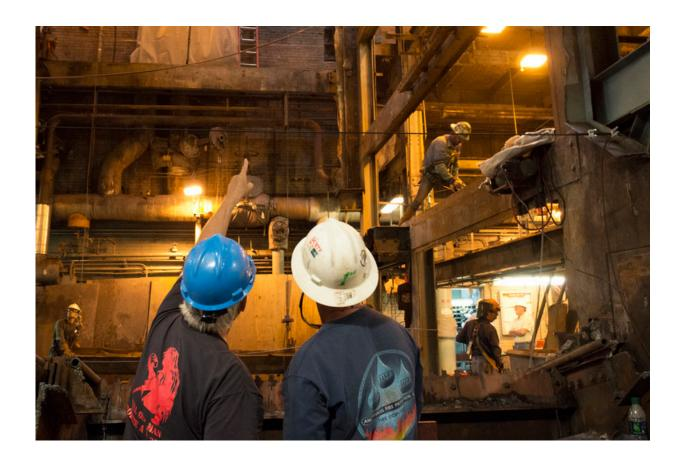
Contractors remove 50-year-old boilers at Penn State's West Campus Steam Plant. The existing boilers in 2014 were deconstructed and removed for the facility's transition to natural gas. A recent study by Penn State researchers found the power plant conversion resulted in no health risks from radon, which is found in natural gas. Credit: Patrick Mansell, Penn State
