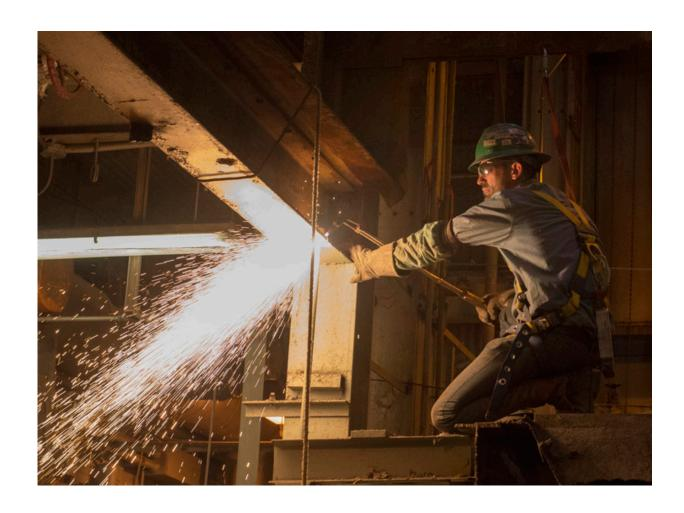
Cutting torches are used to take down support beams during the removal of old boilers from Penn State's power plant in preparation for the facility's conversion to natural gas in 2014. A recent study by Penn State researchers found the power plant conversion resulted in no health risks from radon, which is found in natural gas. Credit: Patrick Mansell, Penn State
