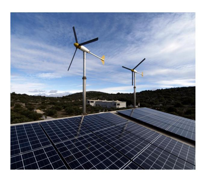
A hybrid wind and solar power system in Zirje, Croatia, includes 2,400 Watts of wind turbines and 4,000 watts of solar cells. Credit: Nenad Kaji via Wikimedia Commons
