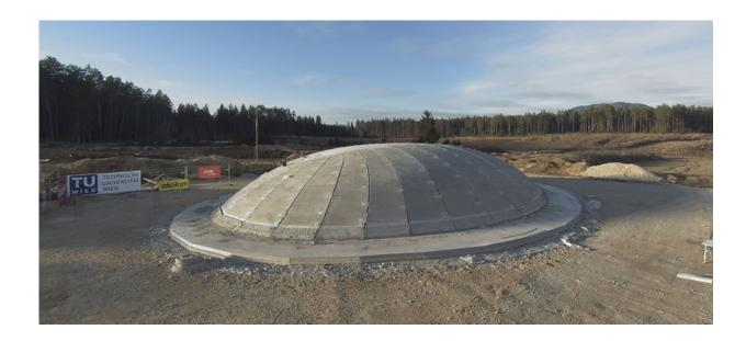
Prepared concrete shell for the application of an additional concrete layer. Credit: Vienna University of Technology
