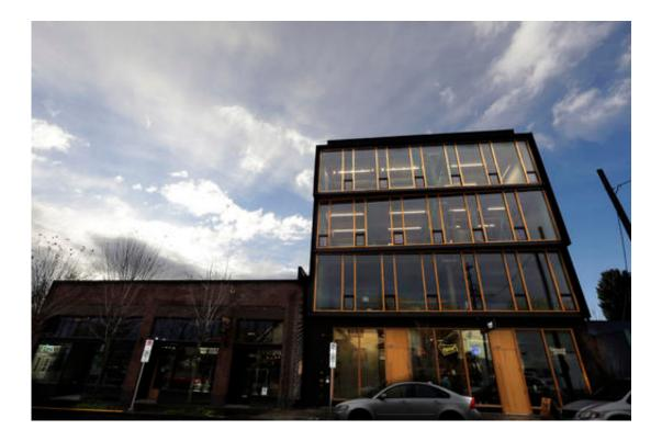
This Nov. 15, 2016, photo shows Lever Architecture headquarters, a four-story all-wood building built using cross-laminated timber, or CLT, in Portland, Ore. CLT is made up of 2-by-4 beams laid out in perpendicular layers that are then glued together to make giant panels. (AP Photo/Don Ryan)
