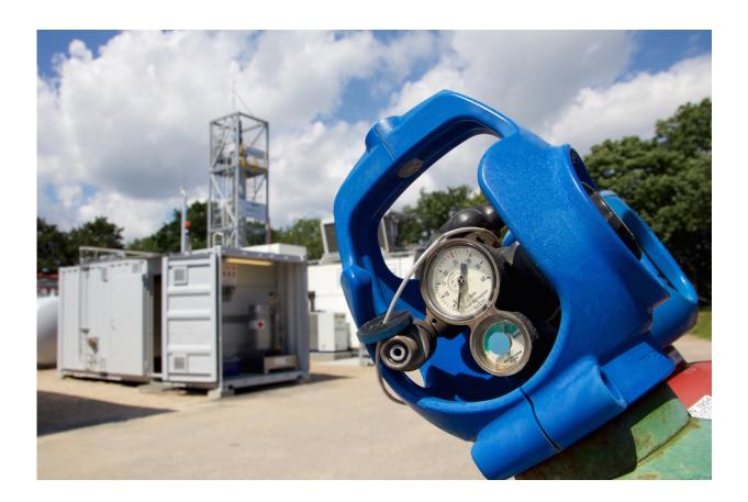
Fully operational since July, Electrochaea's one-megawatt BioCat facility near Copenhagen converts excess electrical power from wind turbines and waste CO2 from the neighboring water treatment plant into methane for the natural-gas grid. Credit: Ronnie Ranch Hedegaard, courtesy of Electrochaea
