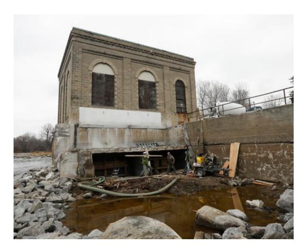
In this Thursday, Nov. 17, 2016 photo, workers close water intakes on a decommissioned hydroelectric powerhouse on the St. Regis River in Hogansburg, N.Y. A century after the first commercial dam was built on the St. Regis River, blocking the spawning runs of salmon and sturgeon, the river once central to the traditional culture of the Mohawk Tribe along New York's northern border is flowing freely again. (AP Photo/Mike Groll)
