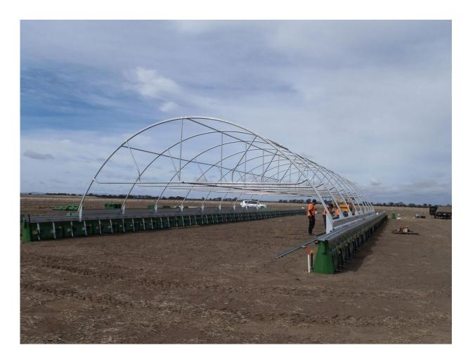
Plastic road barriers, filled with water, and steel arch frames create the skeleton for this portable rainout shelter. Credit: Surya Kant.
