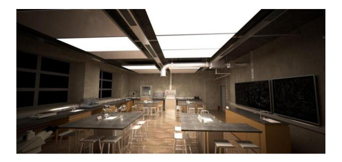
The innovative cooling element reduces perceived temperature in just three minutes. Besides ambient climate control and lighting, the modular system also improves acoustics. Credit: Alexander Buff / Fraunhofer IBP
