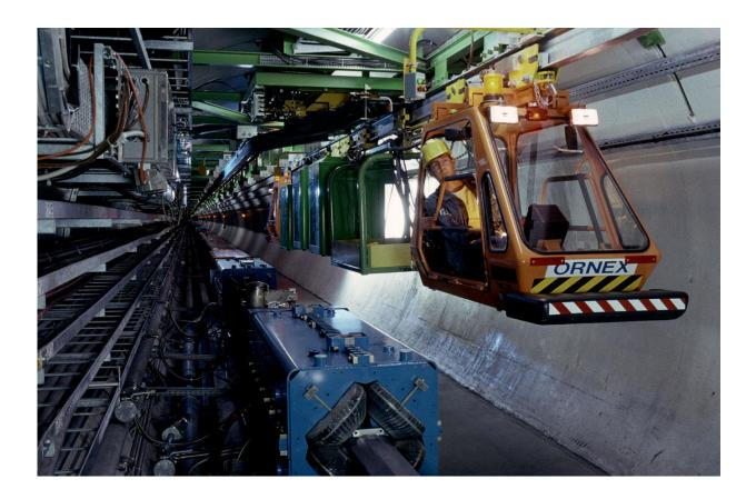
TIM uses the tracks of the former Large Electron Positron (LEP) monorail. This image from 1991 shows the LEP monorail, which carried materials and workers when the tunnel housed the LEP collider. LEP was closed down in 2000 to make way for the construction of the LHC in the same tunnel. (Image: Patrice Loiez/CERN)
