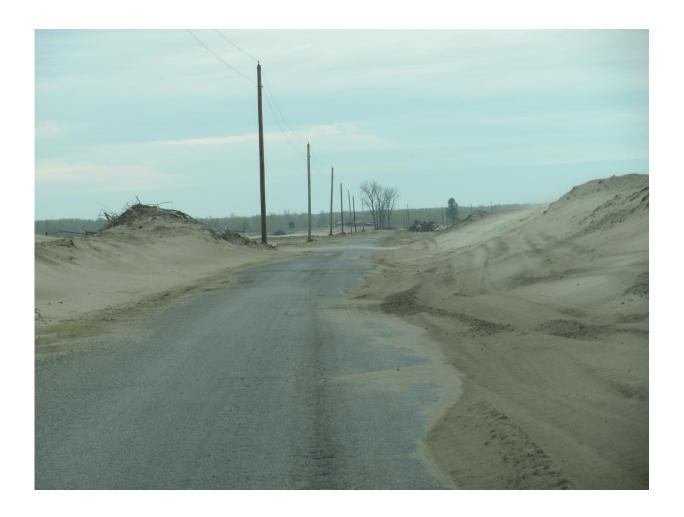
Mississippi River floodwaters deposited many tons of sand on farmland and roads in Dogtooth Bend peninsula when the Len Small levee breached in January of 2016. The sand dunes left behind required graders and snow plows to open the road for local traffic. Credit: University of Illinois
