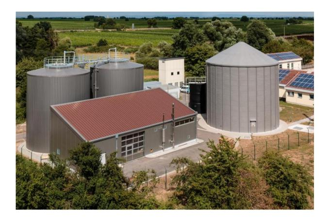
The two-stage high-load anaerobic digestion system in Edenkoben allows the wastewater treatment plant to cope with a higher effluent load during the wine harvest. Credit: Verbandsgemeindewerke Edenkoben
