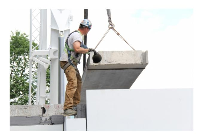
A precast concrete section is lifted into place for a net-zero home built in Edmonton, Alberta, Canada. Credit: MIT CSHub
