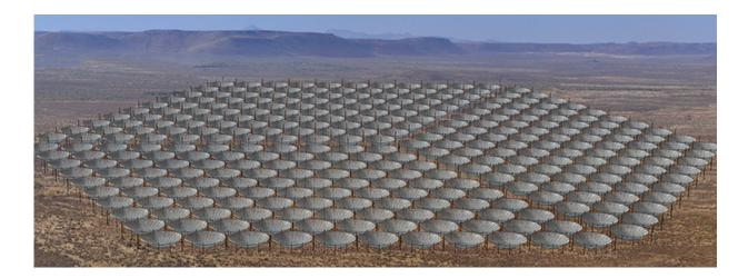
The HERA collaboration expects eventually to expand to 330 radio dishes in the core array, each pointed straight up to measure radiation originally emitted some 13 billion years ago. Twenty outrigger dishes (not shown) are also planned, bringing the array up to 350 dishes total.
