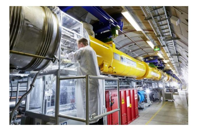
Using a small box as a clean area, technicians make connections between two accelerator modules in the European XFEL tunnel in April. These connections within the modules supply liquid helium to cool the interior of the modules to -271°C, allowing the accelerator's cavities—where the electrons travel—to have superconducting properties. Credit: H. Müller-Elsner/European XFEL
