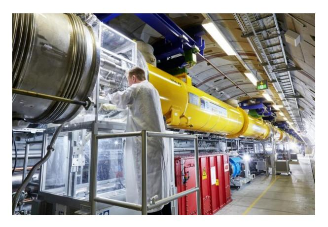
Using a small box as a clean area, technicians make connections between two accelerator modules in the European XFEL tunnel in April. These connections within the modules supply liquid helium to cool the interior of the modules to -271°C, allowing the accelerator's cavities—where the electrons travel—to have superconducting properties. Credit: H. Müller-Elsner/European XFEL
