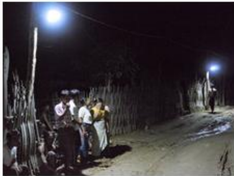
Street lights brightening up the night.
