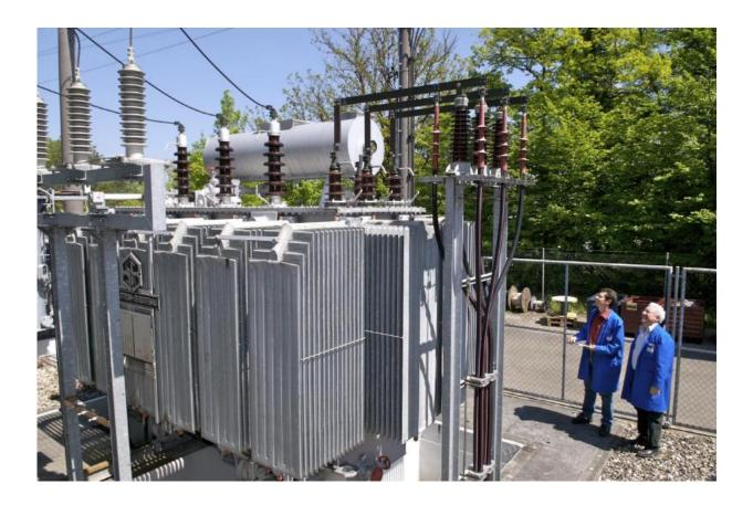
The Paul Scherrer Institute is supplied with electricity from a high-voltage power line at 50 kV. The transformer station shown on the image transforms the electrical voltage to 16 kV before distributing it within the institute. Further transformers situated throughout the institute reduce the voltage to 400 or 230 Volts. Credit: Paul Scherrer Institute/Markus Fischer
