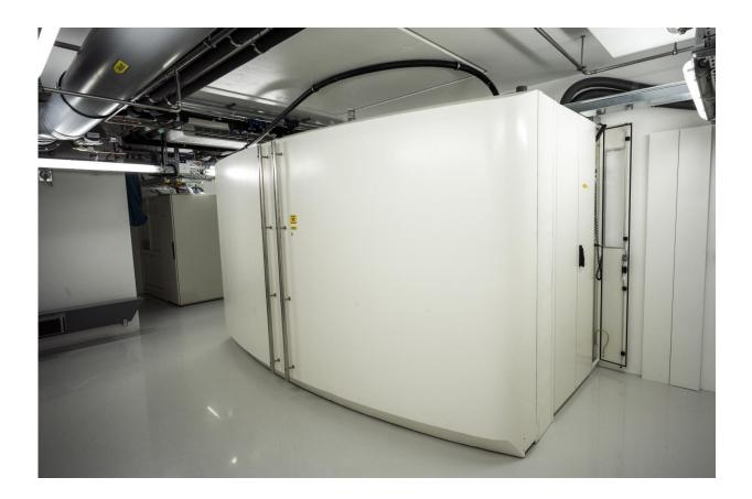
The PETtrace 700S cyclotron with closed radiation shield. Credit: photo/©: Stefan F. Sämmer, JGU
