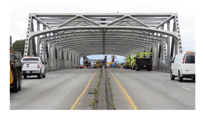
A key factor in the crash was the curved opening of the bridge. The posted height was the maximum in the center, not the lower curved section above the outer lanes, which the truck hit. Credit: Tim Stark
