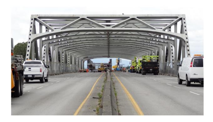
A key factor in the crash was the curved opening of the bridge. The posted height was the maximum in the center, not the lower curved section above the outer lanes, which the truck hit. Credit: Tim Stark
