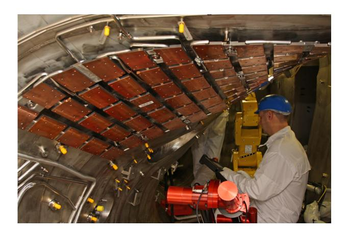
Copper-chrome-zirconium plates for extracting heat, already installed prior to the first round of experiments, will be clad with graphite tiles in the coming weeks. Credit: IPP, Dr. Torsten Bräuer
