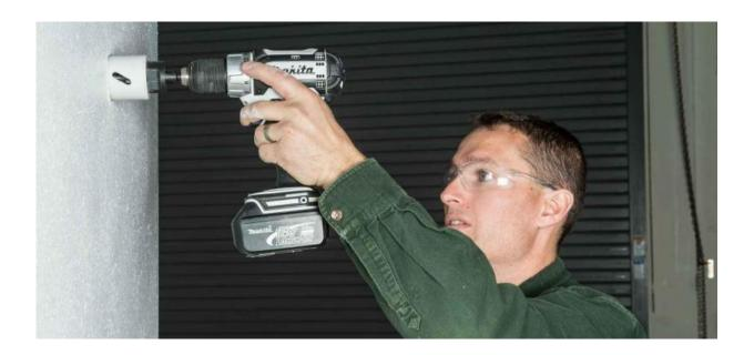
Chuck Booten drills a hole in the wall to mount the EcoSnap-AC. Credit: Dennis Schroeder
