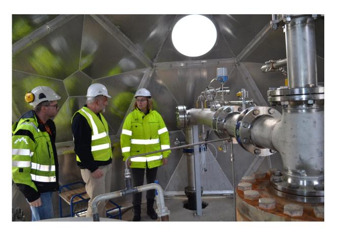
Engineers and scientists have designed a system to pump volcanic gases including carbon dioxide back into the earth, where the CO2 turns into a solid. Left to right, engineer Magnus Thor Arnarson, Lamont-Doherty Earth Observatory hydrologist Martin Stute and project leader Edda Sif Arradotir of Reykjavik Energy inspect the downgoing piping system. Credit: Kevin Krajick/Lamont-Doherty Earth Observatory
