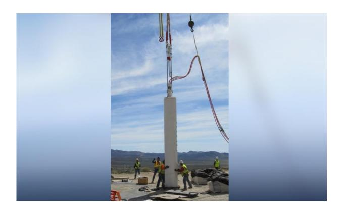
Workers at the Nevada Nuclear Security Site are shown lowering the 25-footlong Source Physics Experiment (SPE-5) canister into the borehole to its center depth of 76.5 meters or about 250 feet.
