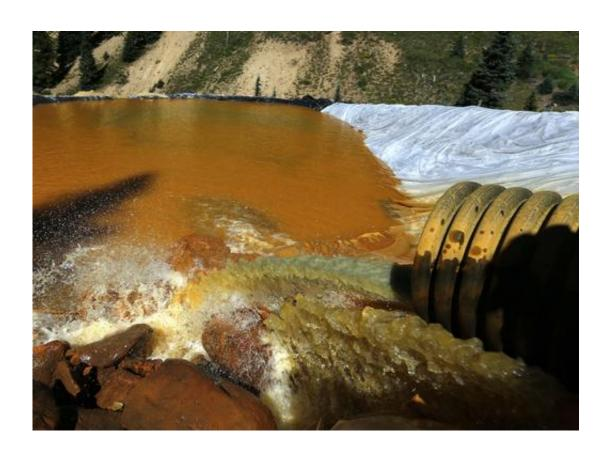
In this Aug. 14, 2015 file photo, water flows through a series of retention ponds built to contain and filter out heavy metals and chemicals from the Gold King mine chemical accident, in the spillway about 1/4 mile downstream from the mine, outside Silverton, Colo. Researchers who studied a river in Colorado after a massive mine spill say runoff from fall storms kicked up the levels of some contaminants in the water but not others. (AP Photo/Brennan Linsley, File)
