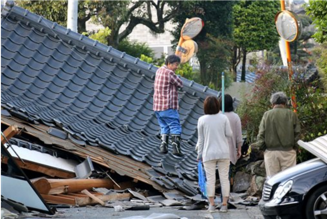
Residents look for an access to their home on the road which is blocked by a collapsed house, in Mashiki, Kumamoto prefecture, southern Japan Saturday, April 16, 2016. A major quake shook southwestern Japan, barely a day after another quake hit the same region. (Naoya Osato/Kyodo News via AP)
