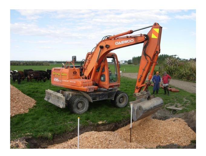
Bioreactor design varies, but they are typically large trenches filled with wood chips. Credit: Brandon C. Goeller, University of Canterbury, Christchurch, New Zealand.
