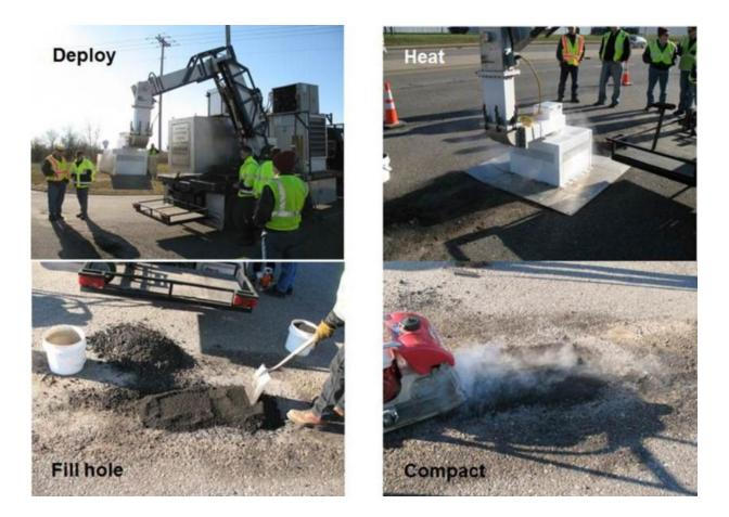
Steps to an effective microwave pothole repair. Credit: Zanko et al., 2016, CC BY-ND
