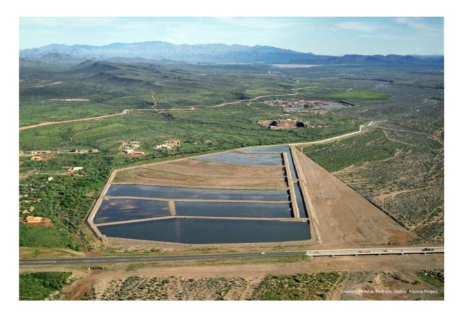
The Agua Fria Water Recharge Facility, a spreading basin in Arizona. Water collected by the facility percolates into the aquifer below it. Credit: Central Arizona Project
