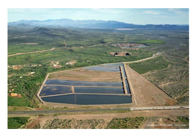
The Agua Fria Water Recharge Facility, a spreading basin in Arizona. Water collected by the facility percolates into the aquifer below it. Credit: Central Arizona Project
