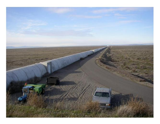
Exterior of a section of one of the arms of the LIGO interferometer on Hanford Reservation in Washington. Credit: Umptanum, CC BY-SA
