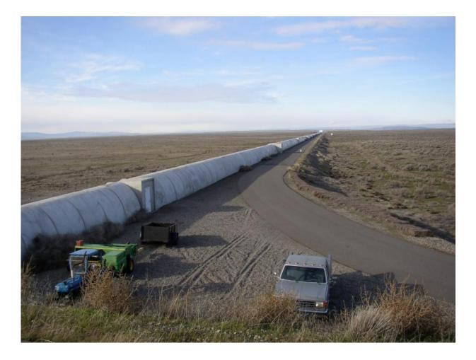
Exterior of a section of one of the arms of the LIGO interferometer on Hanford Reservation in Washington. Credit: Umptanum, CC BY-SA
