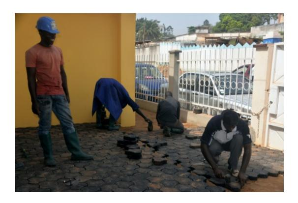
Workers pave the ground with recycled cobblestones made of plastic waste, in Yaounde, Cameroon
