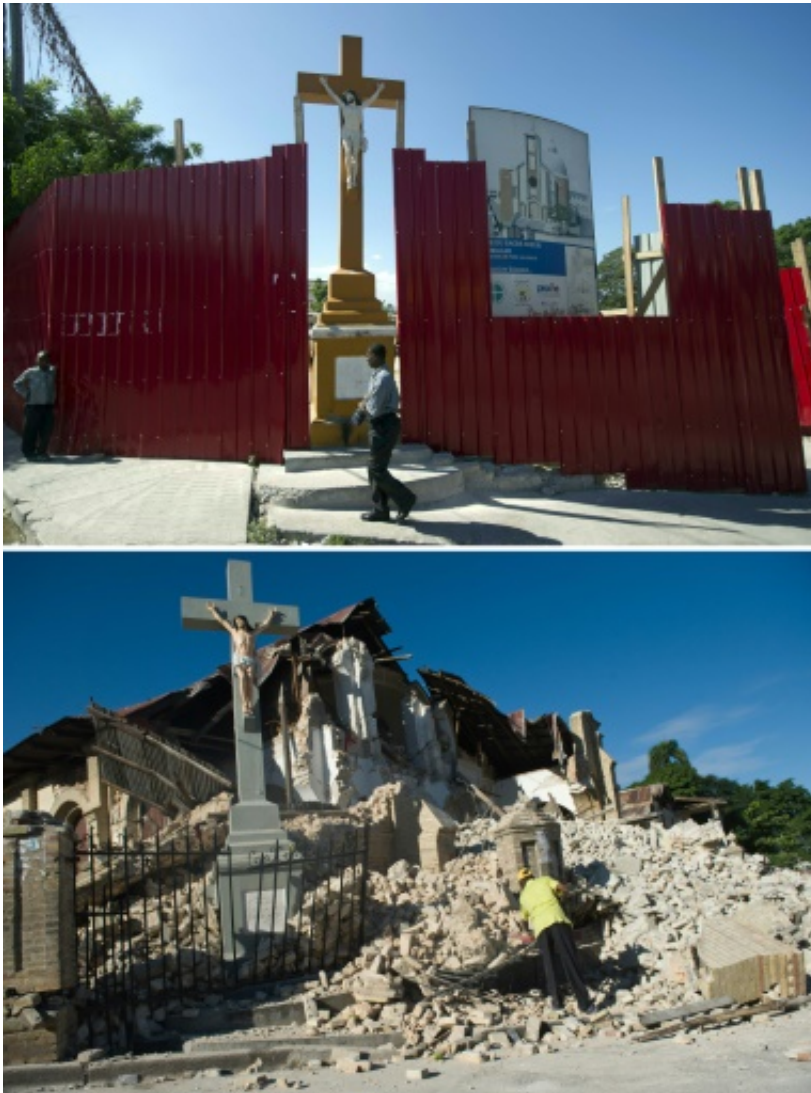
The Sacre Coeur Church in Port-au-Prince, on December 29, 2014 (top) and the church on January 14, 2010, two days after it was destroyed by the earthquake (bottom)
