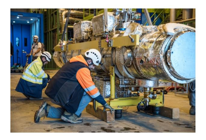
On 12 January, members of the team working on CERN's year-end technical stop prepare to install one of the LHC's new beam absorbers. The six-metre-long component will be lowered 100 metres into the LHC ring.
