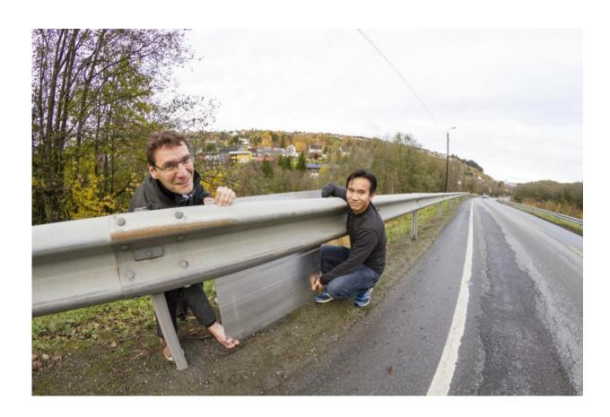
Standard guardrails in Norway are often installed where the ground falls away from the roadside. Houses that are to be screened from noise in such locations usually lie somewhat lower than the source of noise. Taking this as the basic situation, SINTEF scientists Dirk Nolte (left) and Nguyen Hieu Hoang investigated how aluminium noise-barriers could be directly mounted on guardrails. Credit: SINTEF/Thor Nielsen
