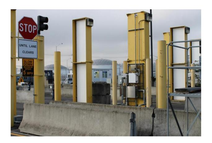
Radiation portal monitors like these alarm less frequently on cargo materials such as tile or granite that may contain non-threatening, naturally occurring radioisotopes thanks to a new approach developed by PNNL, which emphasizes the use of selective energy-sensitive algorithms.
