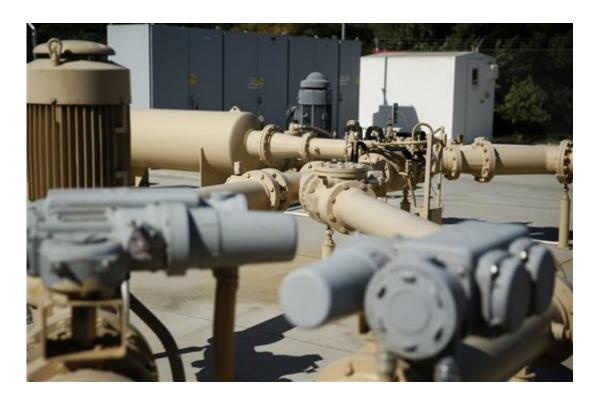
In this Sept. 17, 2015 photo, pipes are used to blend water from a well at the location with treated water from other sources in Modesto, Calif. The city of Modesto, with a half-million residents, recently spent more than \$500,000 to start blending water from one contaminated well to dilute the uranium to safe levels. The city has retired a half-dozen other wells with excess levels of uranium. (AP Photo/John Locher)
